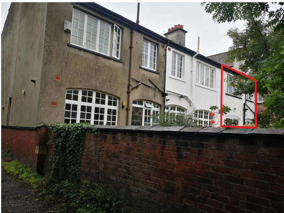
The rear of properties on Cotton Lane (24-28) number 28 is highlighted in red
