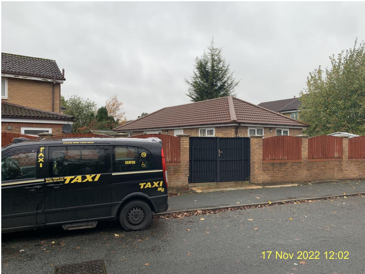
Photograph 1 Single storey dwellinghouse as viewed from Montcliffe Crescent
