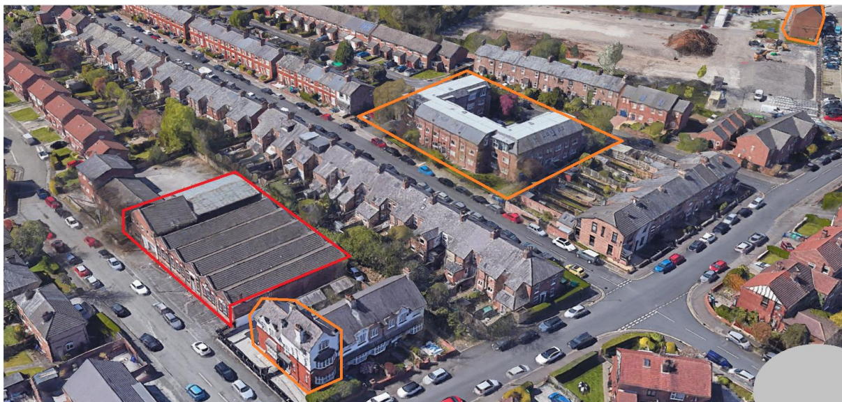
Application site (edged red) and nearby properties with three storeys edged in orange
