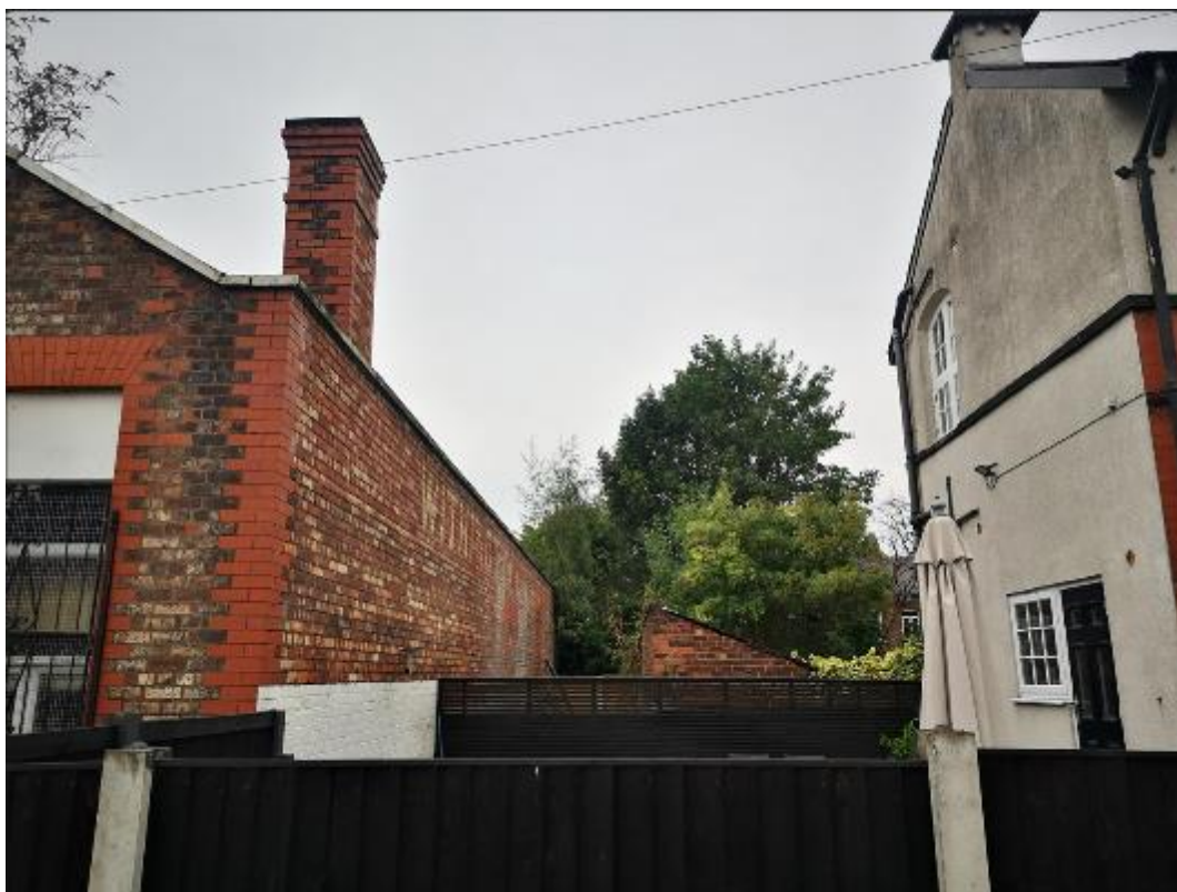
Photograph of relationship between the existing laundry building on the left and the rear gable wall of number 30 Cotton Lane to the right
